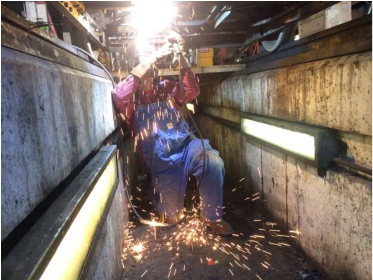
Cliff welding the cross-brace under the A-6
